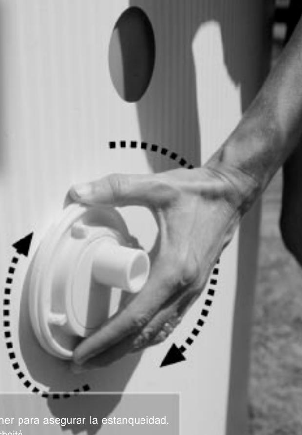
In order to ensure leak-tightness seal (10) must perfectly fit against the liner.
