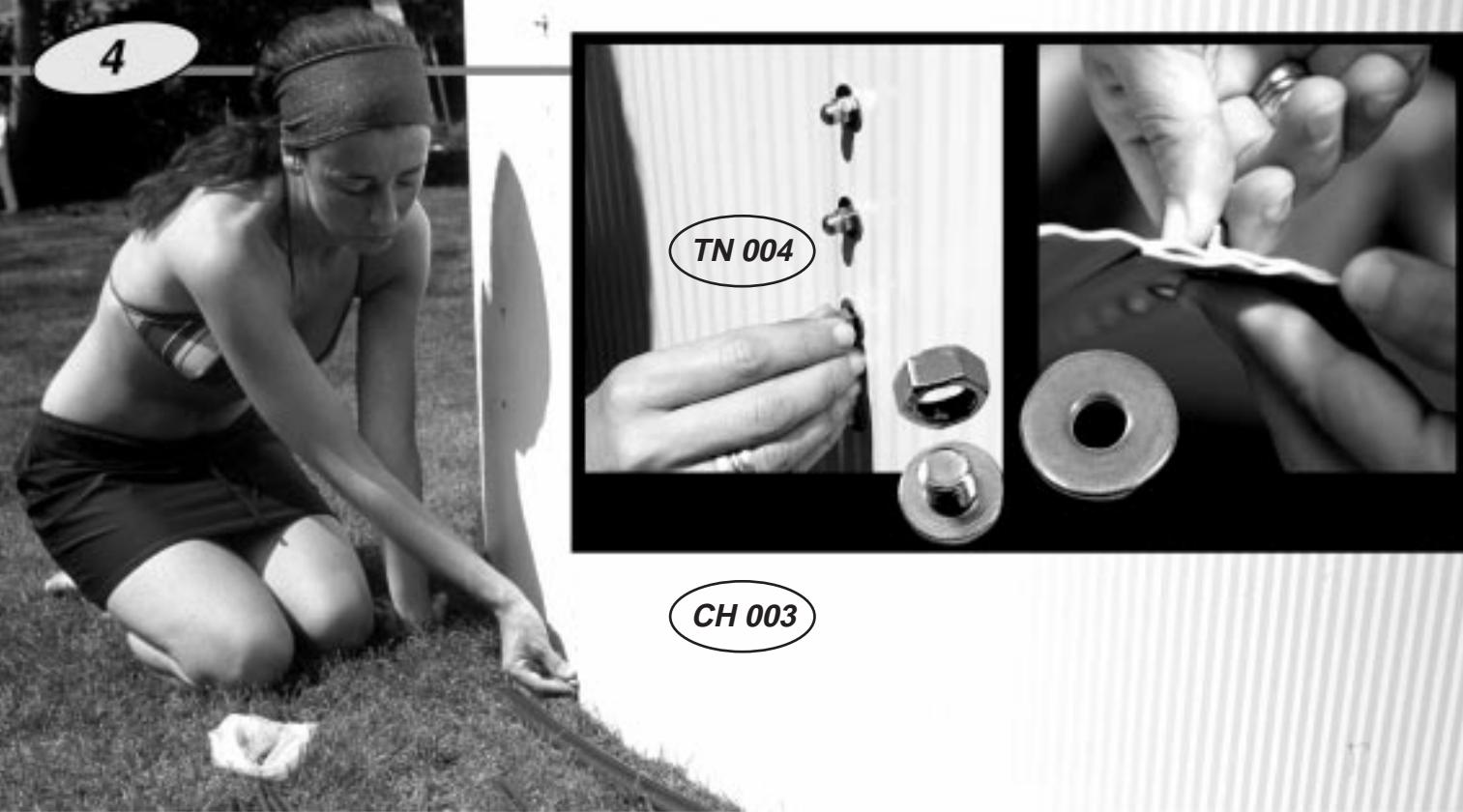
**With** the sheet joined up, check that all the sections are well seated to cut the lower closing section to the right length
